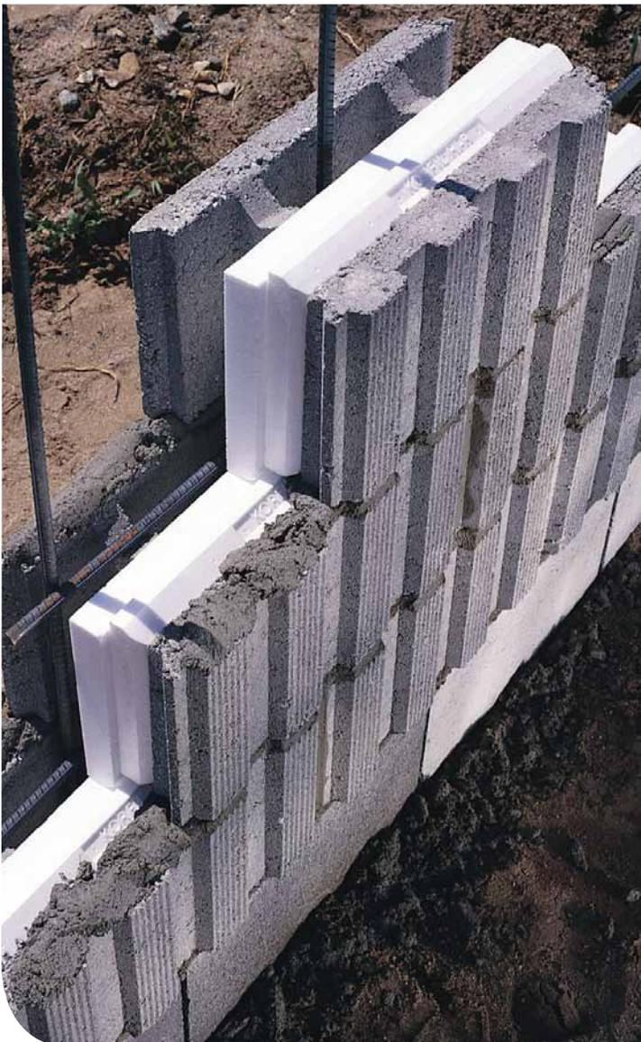
Depending on the materials and type of wall assembly selected, performance criteria can be specified to an exact degree. Designing for energy performance that exceeds minimum requirements is most easily achieved by adding foam plastic insulation.
